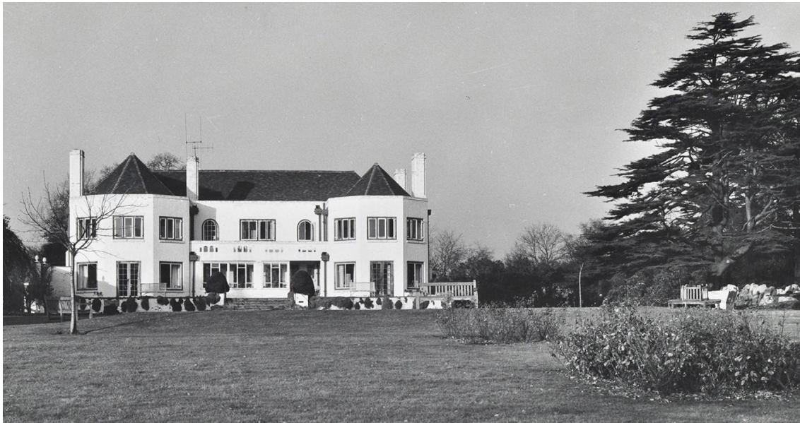
4.5 Kinellan in the 1960's as 33 Camp Road, from the rear (London Metropolitan Archives, City of London [Collage: the London Picture Archive, ref SC_PHL_02_0178_64_282 (No. 176925)])
